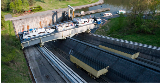
Marvel of modern engineering – the St-Louis / Arzviller Boat Lift.
